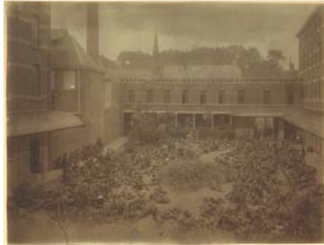
View of the courtyard
